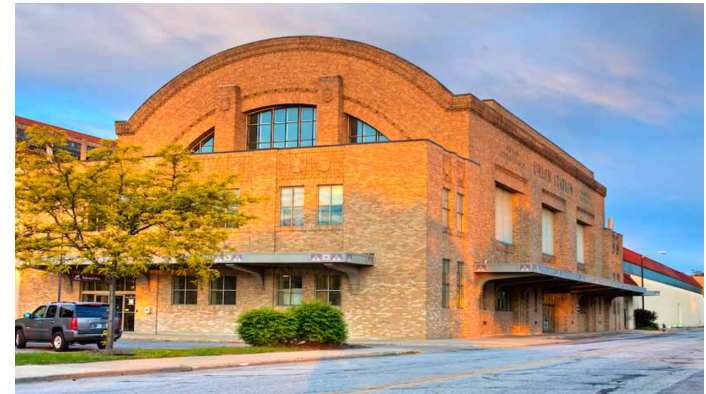
CRC HPC Center (old Union Station)
